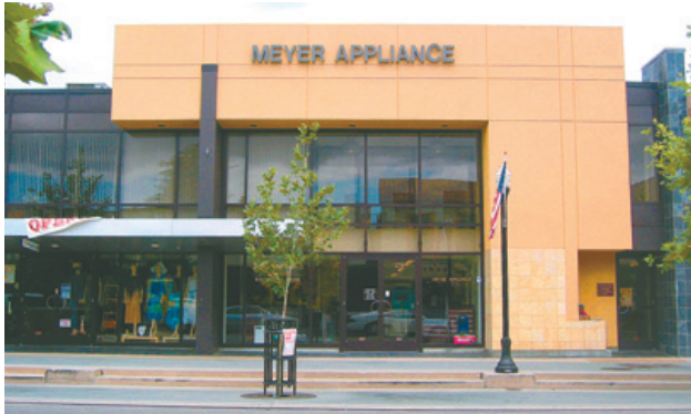
The Mountain View store after a $4,000,000 remodel
